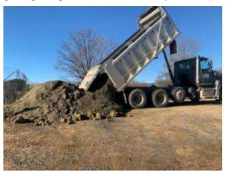
Two trucks later, we were ready to start spreading out all this material to create a smooth surface that will drain. Greenhouses are very wet environments, and it is very important to have a good, level, well-draining floor for the structure. Now that we have 12 years experience with one, we have a pretty good clue about what works!
