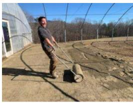
After we got the rock dust spread, leveled, and packed it was time to cover the surface with landscape fabric. Again, this was a precise operation. But we were able to get 30 feet of fabric installed before we had to prepare for an inch of rain. :- (
