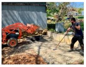
Tamping and leveling, tamping and levelling... a little bit at a time creates a good foundation.
