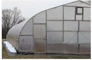
A nice thing about this weather is that it has given us the opportunity to get lots of inside work done. Ray and Jonny have been working on getting the greenhouse buttoned up more. The north wall of the structure has always needed to be insulated and we started tackling that project. Instead of a single layer of plastic, the wall will have 2 layers of plastic with foam insulation sandwiched in between.
